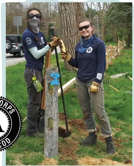
Installing split rail at Mill Pond Overlook
